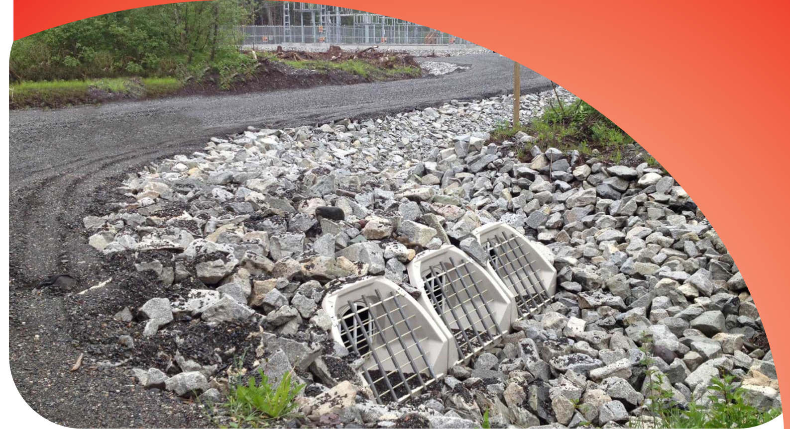
Aprons are available for high erosion wash-out conditions
